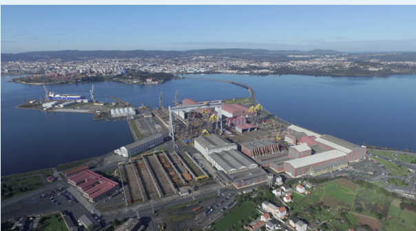
Fene Yard, Spain (1.000.000 m 2 )
