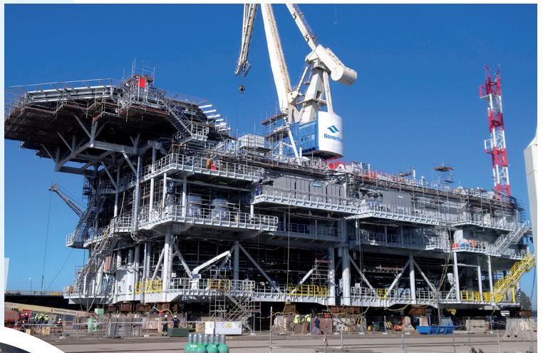
5000 t Wikingier Substation Topsides under construction Puerto Real (Spain)
