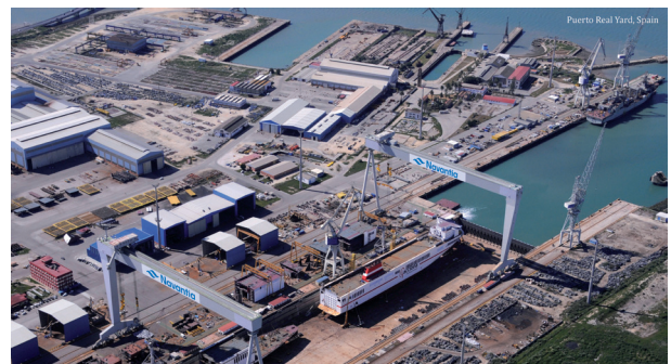
Puerto Real Yard, Spain (1.200.000 m 2 )
