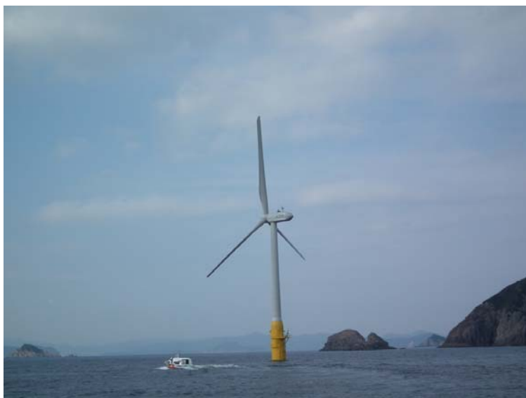
Fig1. GOTO FOWT floating offshore wind turbine demonstration project, Hitachi 2MW on the spar type floater, Courtesy of MOE
