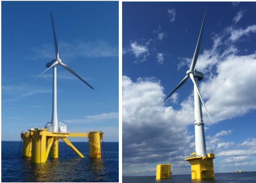
Fig2. FukushimaFORWARD floating offshore wind farm demonstration project, Hitachi 2MW & MHI 7MW on the semi-sub type floater, Courtesy of METI
