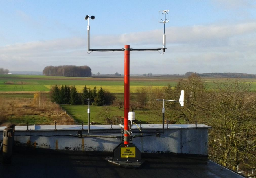
Figure 2: mast installation in Choczewo pilot site
