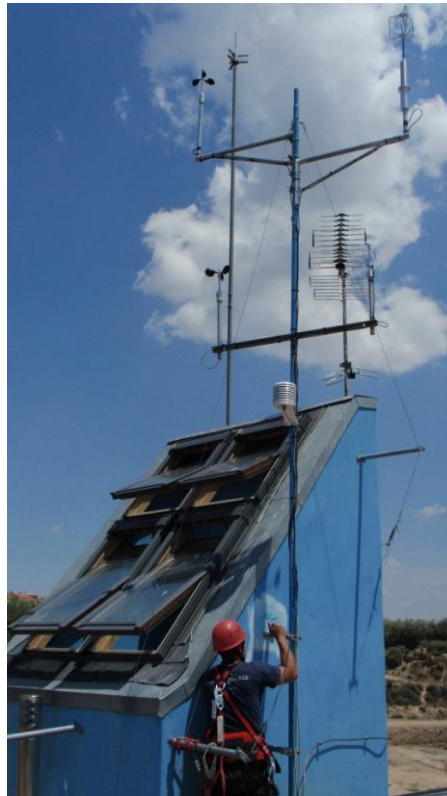
Figure 5: mast installation in Zaragoza pilot site
