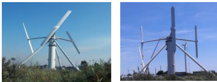
Fig.1. Two NENUPHAR's onshore prototypes: different rotor configurations were tested (twisted and canted blades and straight vertical blades), both for a period of approx. 1 year
