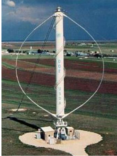
Figure 4. Photograph of Sandia 34m VAWT
