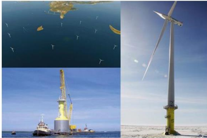
Frozen... The 2.3MW pilot turbine (right) is sited off Finland, testing the arctic weather conditions on the turbine and steel cassion foundations (left) ahead of installing the country's first commercial offshore project (top)
