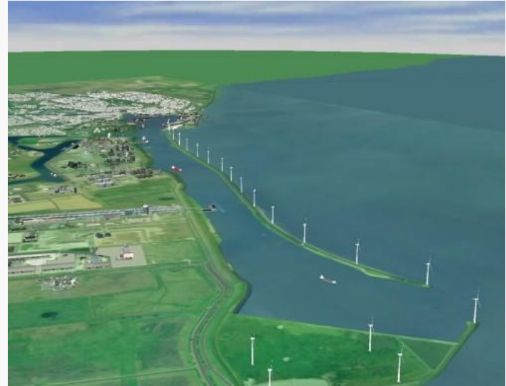
Eemshaven (Netherlands) Partnership with Eneco
