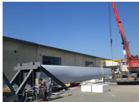
Figure 8: Photograph showing strut calibration
