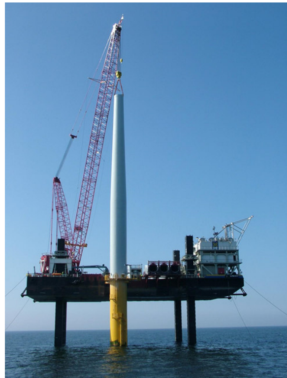
Construction of an offshore WTG
