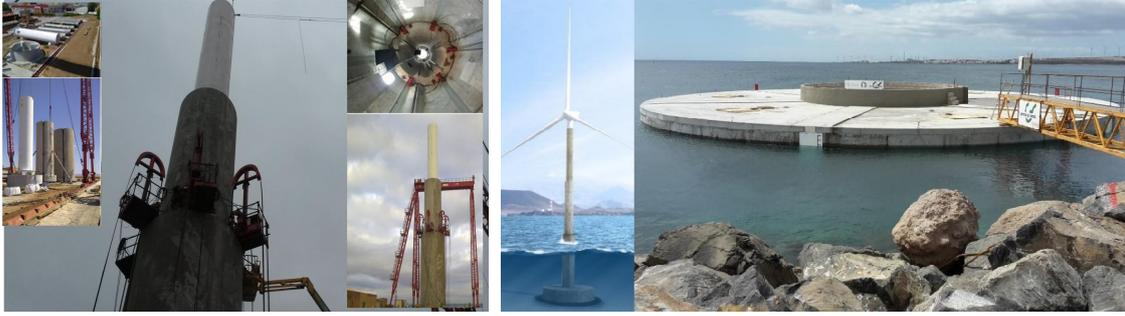
Figure 1. ELISA/ELICAN. Telescopic tower built in Daganzo (Madrid 2014) (left) and GBS under construction in the Canary Islands (Sept-16) (right).
