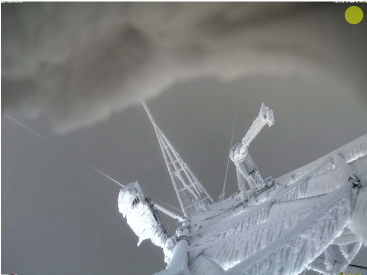
Fig. 4: Camera image on 13/02/2015 with high icing intensity
