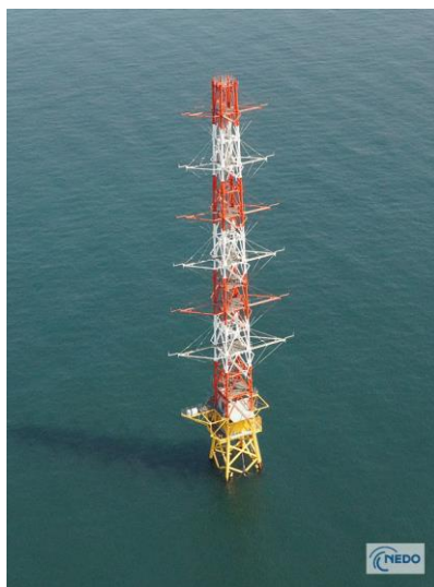
Figure 1: NEDO offshore meteorological mast off Kitakyushu City, Fukuoka Prefecture (from NEDO website)
