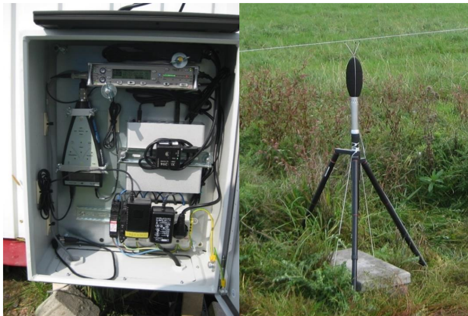
Figure 2: Permanent sound measuring station; left: used enclosure with sound recorder (upper device), sound level meter (greenish device on left side) used as preamplifier, a hard disk drive (silver box on the right side) and some power supply equipment at the bottom; right: used weatherproof microphone unit on a stand
