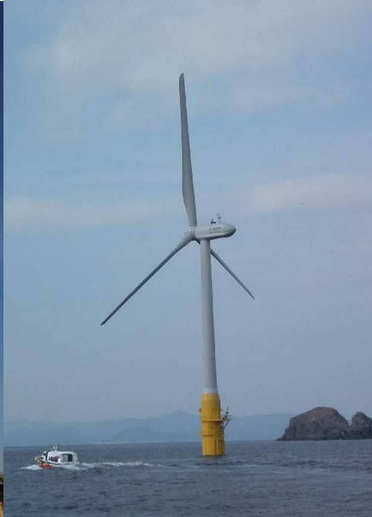
Hitachi Co. 2MW, downwind, geared
