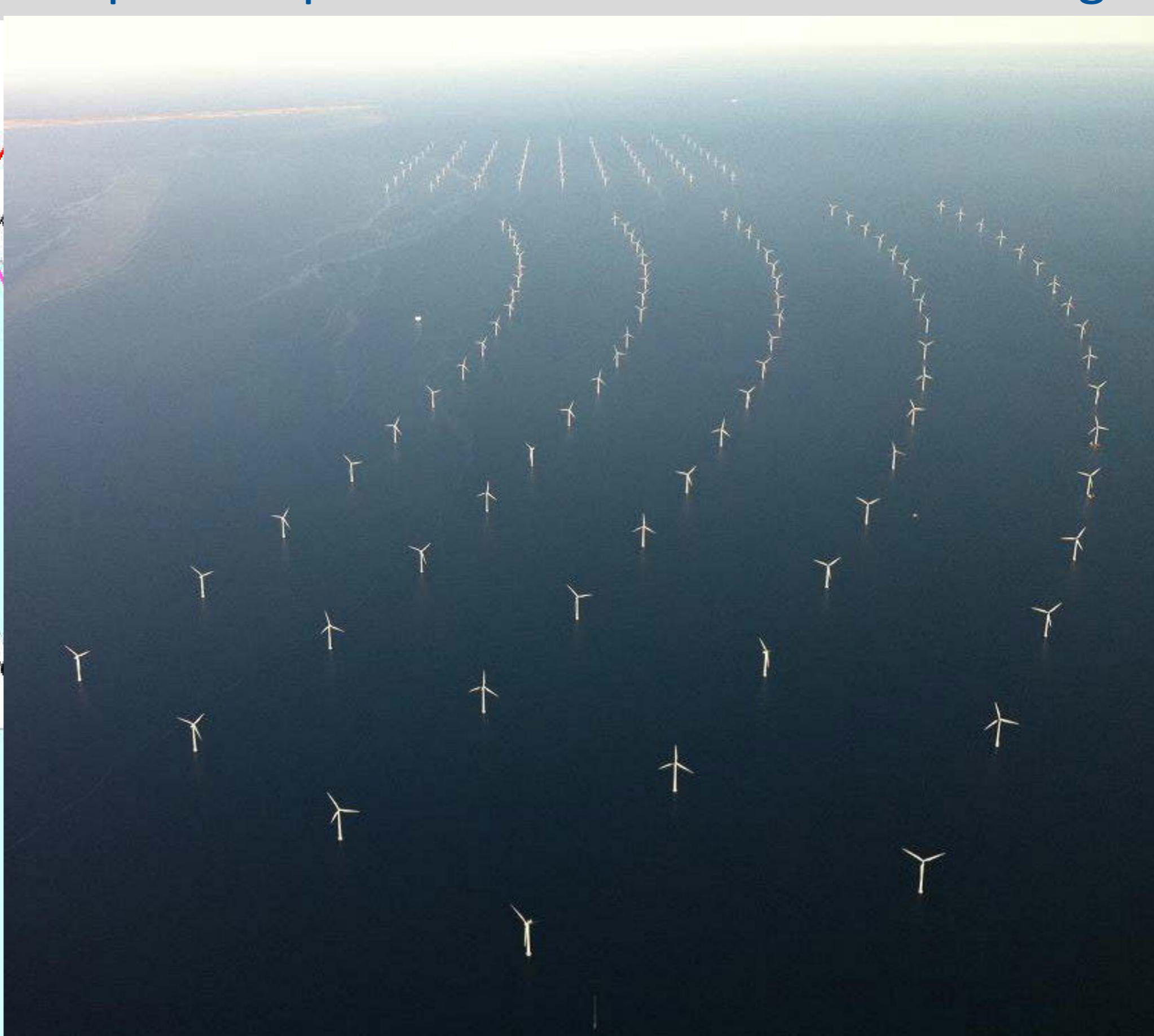
Fig. 2 Rodsand 1 and 2 OWPP south to Denmark East.
