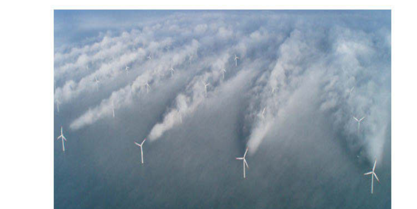
Figure 3: Example of "wake effect" in a wind farm offshore. Overlap of a wake effect with a WT rotor. This is a very important factor in the WT placement.
