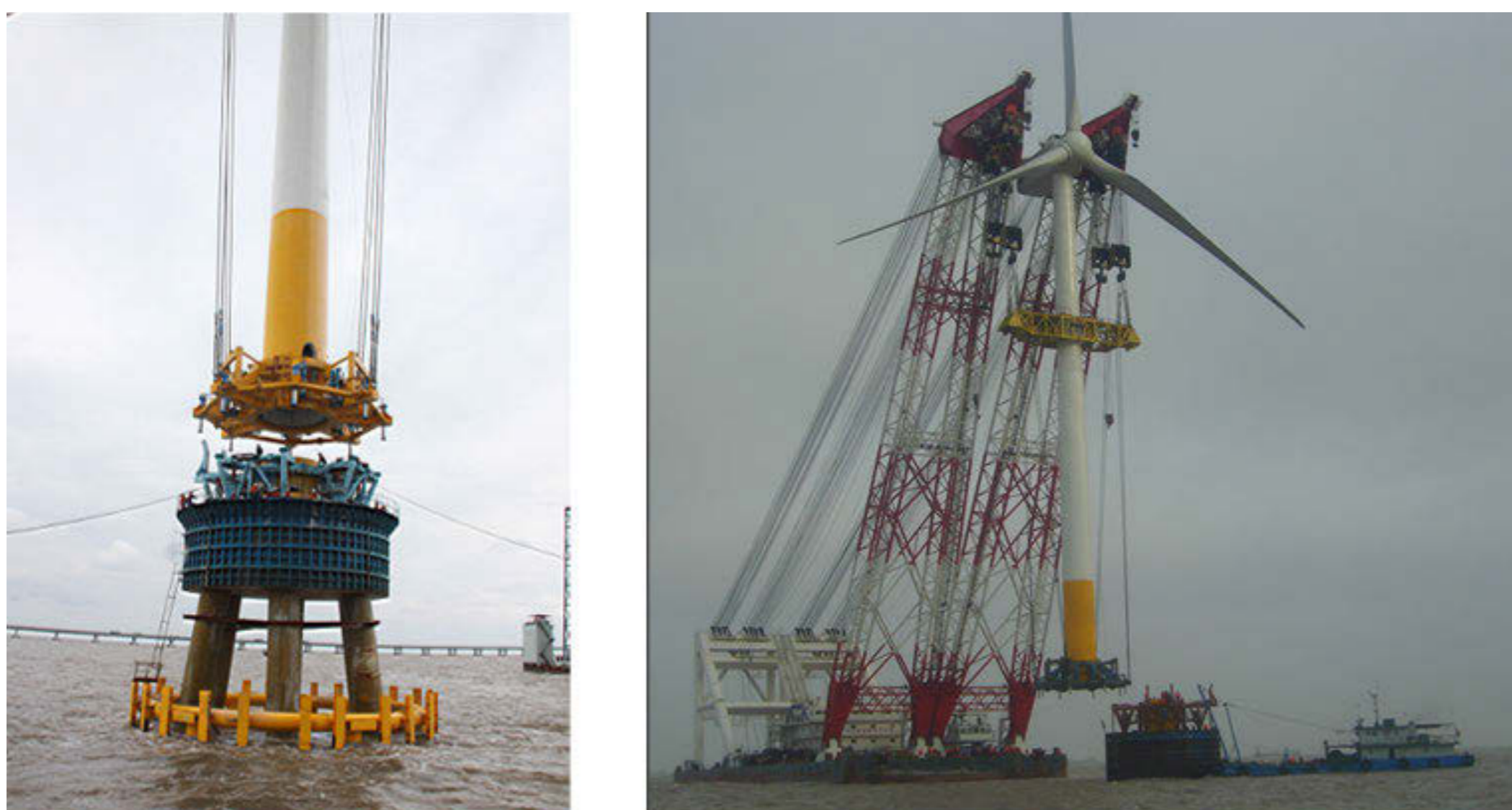
Fig. 1 New foundation Fig. 2 Installation of fully assembled wind turbine (courtesy Yifeng Lin)
