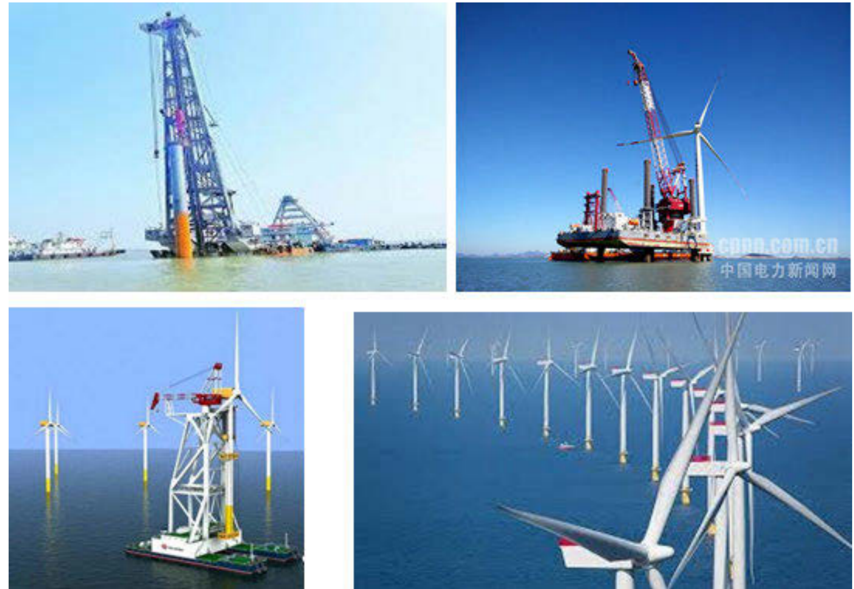
Fig. 4 Installation of Nanri 4MW wind turbine and an aerial view of the wind farm (courtesy CPNN)
