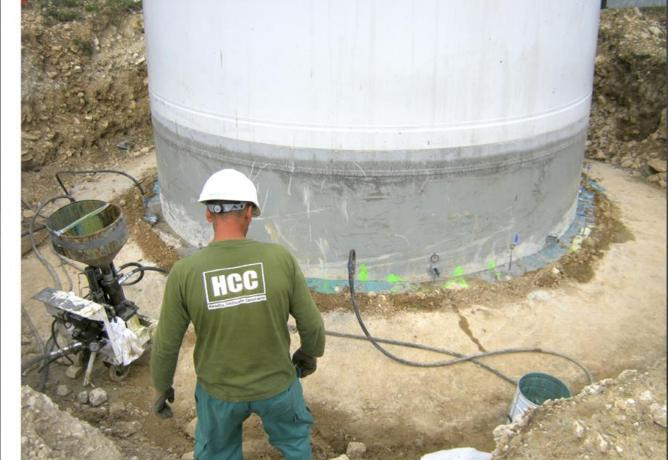
The aim was to return the monolithic concrete fractured under the flange and encapsulate the ferrule on its pedestal, with a strong and elastic material, minimizing the movements and ensuring the durability of the repair.
