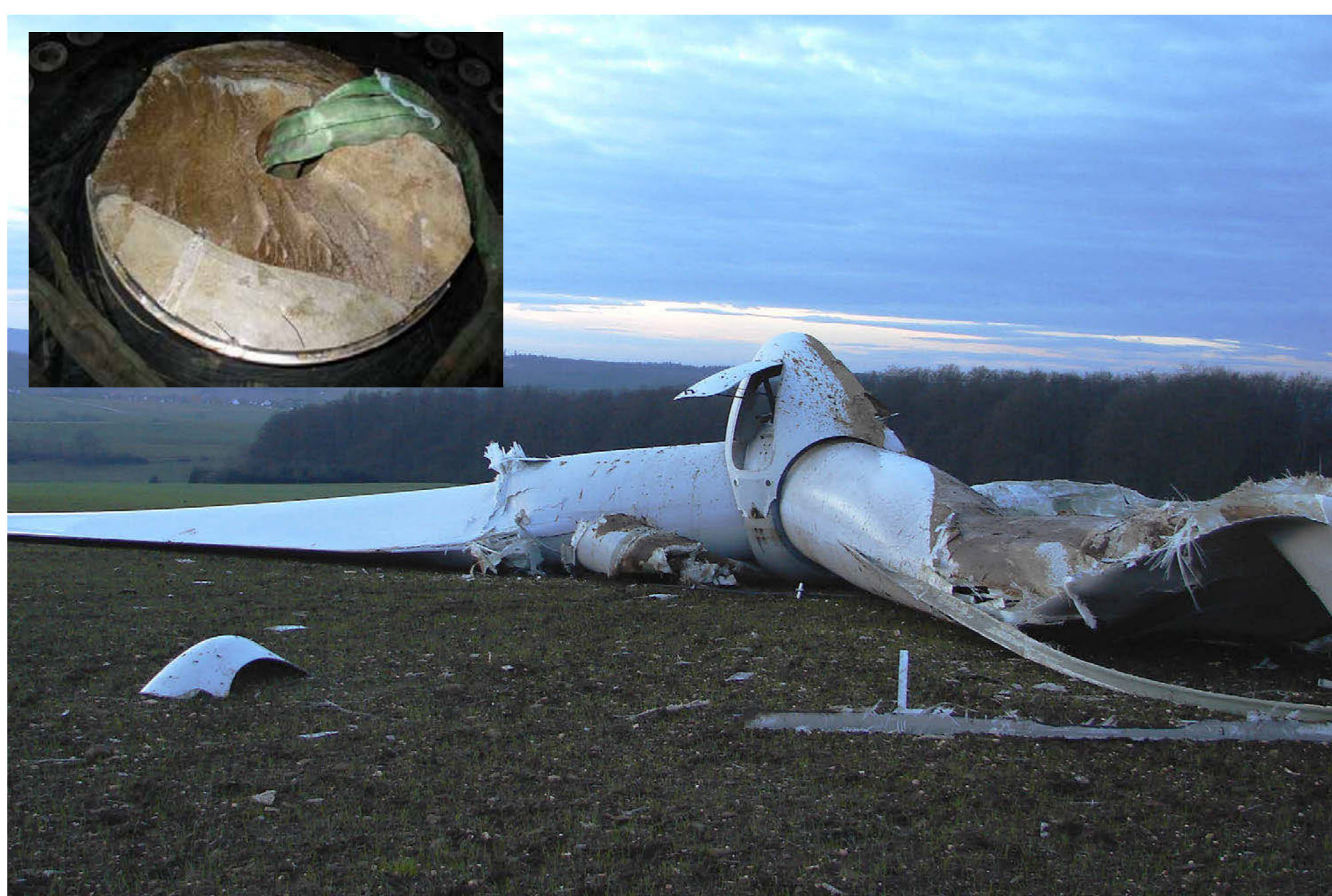
Figure 1. Fatigue can cause severe damage
