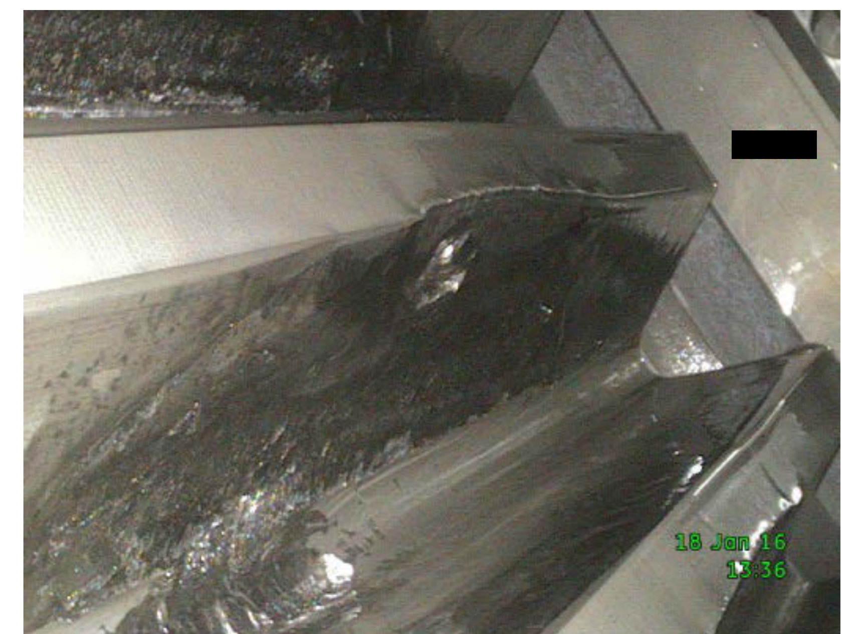
A planet ring gear deformed and broken
