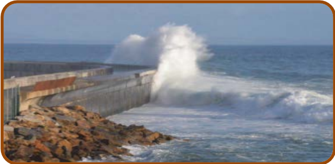
Provide sufficient weight to withstand wave forces
