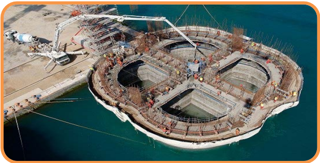
Cellular structures – so they are self-buoyant
