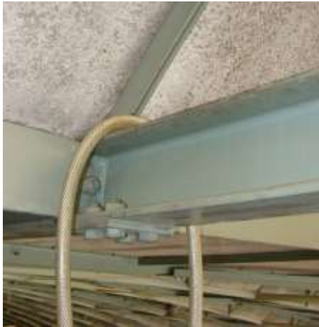
Steel sling at joint.
