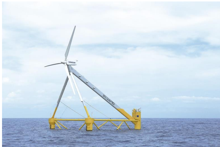
X30 Floating Wind Prototype installed in the Canary Islands.
