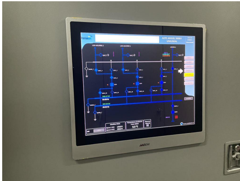
General one-line diagram on Touch Screen
