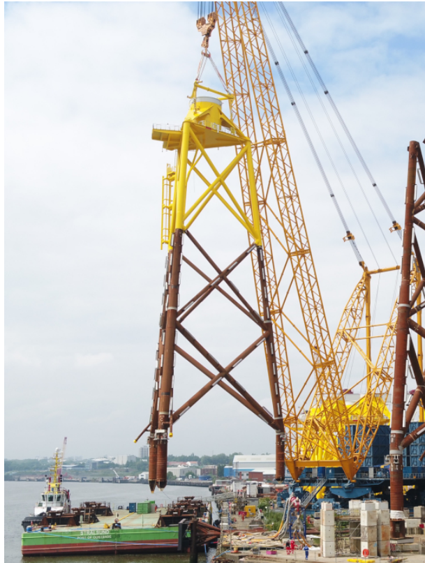
Photo 1: REM-B Hydraulics remote-controlled hydraulics powerpacks for lifting 1000 tonne, 85m high, offshore wind turbine bases.
