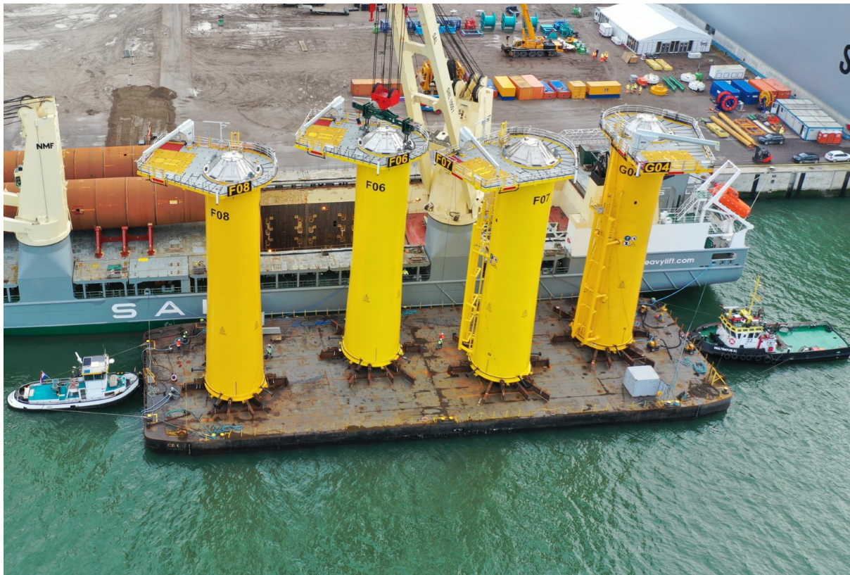
Photo: Transition pieces for the Saint-Nazaire Offshore Wind Project being loaded on a barge at the production facility of Smulders in Hoboken Belgium.
