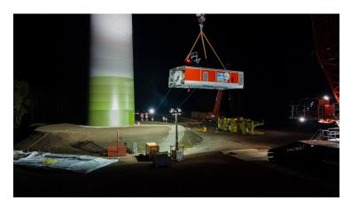
A crane is hoisting the E-nacelle, weighing about 80 tonnes, to a hub height of 166 metres.
