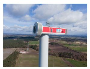
A plug-and-play design provides for the quick installation of the E-nacelle at the construction site.
