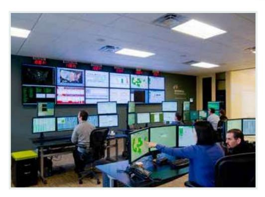
Iberdrola Renewables is using OPC as the communications protocol, along with other protocols, to pull data from the various PLCs. Wind farm applications often use OPC™ and the KEPServerEX™ driver to communicate seamlessly with diverse systems. Iberdrola uses PcVue's OPC Data Access Client and the OPC DA XML Client for exchange of real-time data with communication servers, plus the OPC DA Server to facilitate data exchange with third party applications.
