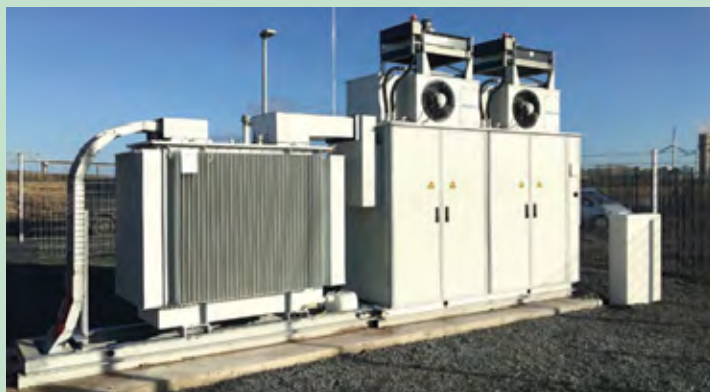
Figure: Battery storage power plant, Wind to Gas Energy Photo: Wind to Gas Energy GmbH & Co. KG 32
